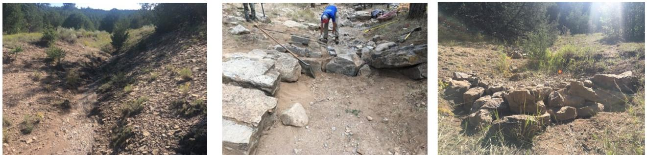
**Figure 15. Bank erosion (left), structure installation (center), and installed structures (right). Photo credit: Rocky Mountain Youth Corps/Stream Dynamics, 2019**
