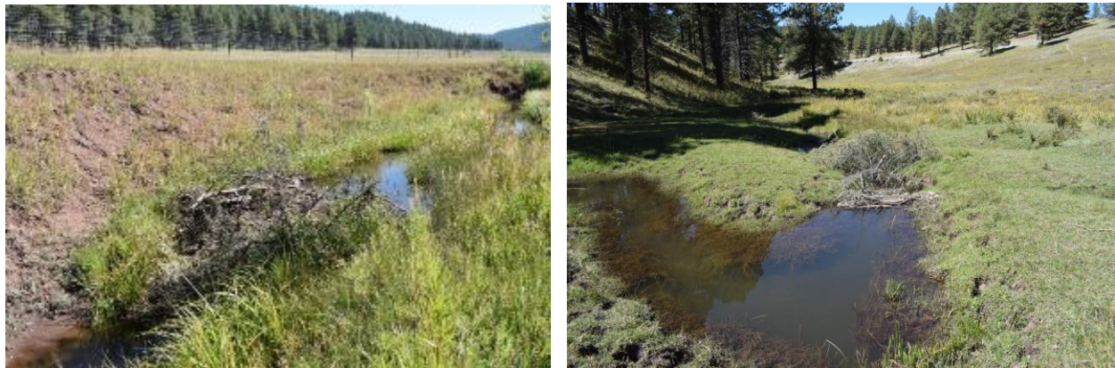
Figure 23. Images showing work completed. Image (left): BDA installation, with exclusion fencing at top of slope; Image (right): An installed BDA, demonstrating the additional ponded area behind BDAs
