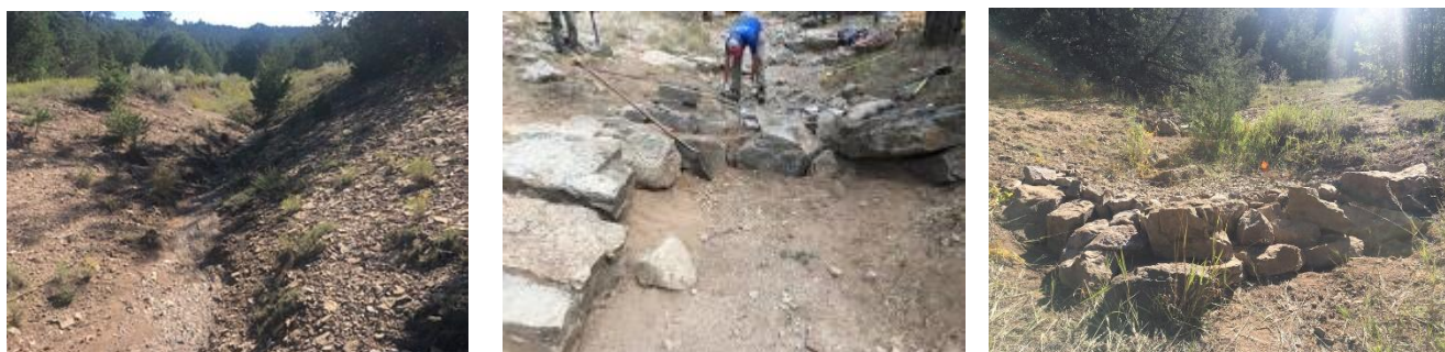
Figure 19. Bank erosion (left), structure installation (center), and installed structures (right).
